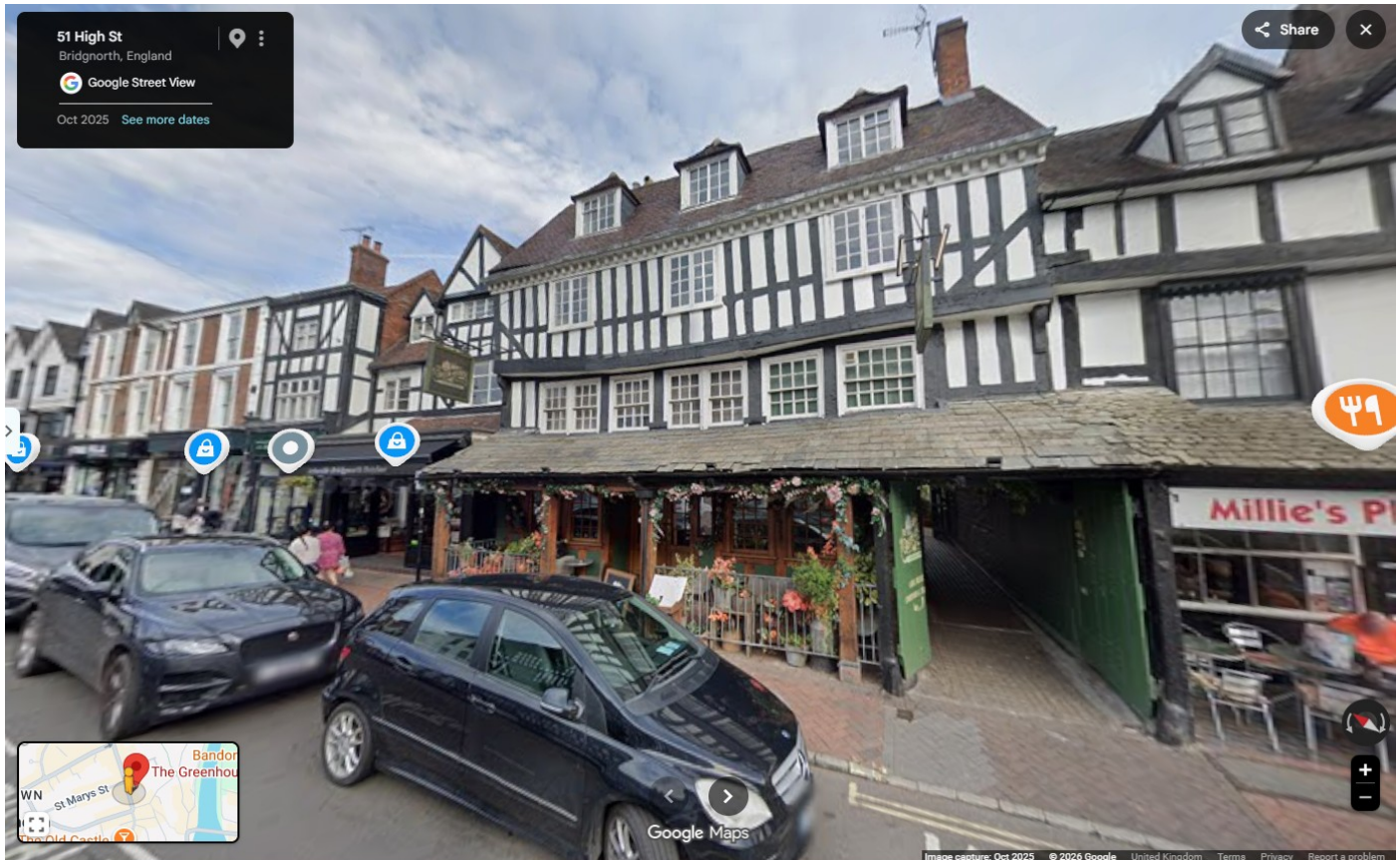
- Front view of the premises -
